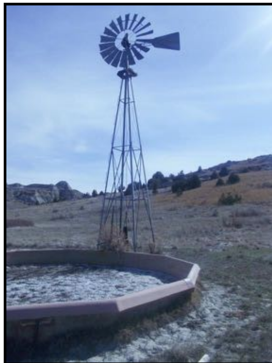
Figure 25: Active Water Tank between log points M1 and M2
